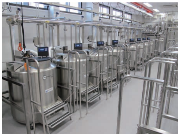
Figure 1. Cryogenic storage system. Liquid nitrogen tanks are monitored for 24 hours and are refilled automatically.
