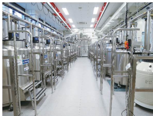
Figure 2. Cryogenic storage system. Liquid nitrogen tanks are monitored 24 hours a day and are refilled automatically.
