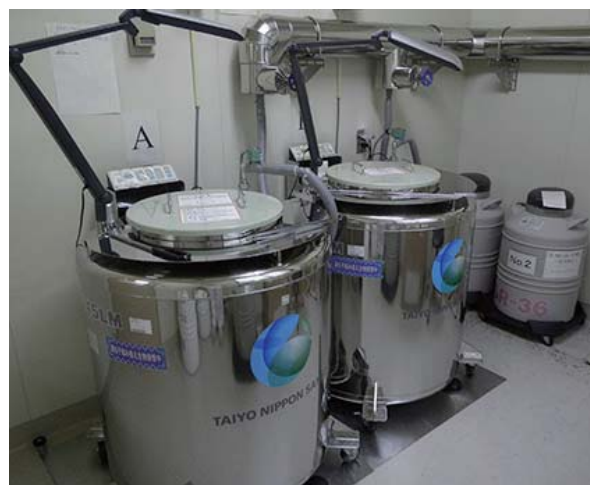
Figure 4. Liquid nitrogen tank.
