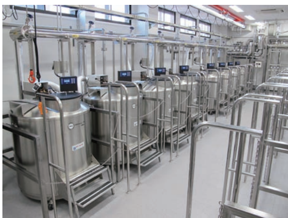
Figure 2. Cryogenic storage system. Liquid nitrogen tanks are monitored 24 hours a day and are refilled automatically.
