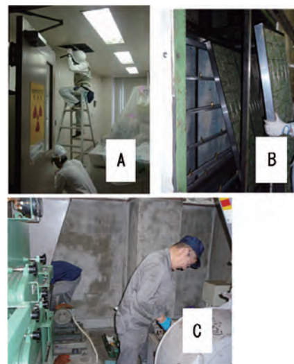
Figure 3. Repair work on air supply & exhaust system at CFBI-branch A: The room re-heaters were replaced. B: The air supply system's eliminators were replaced. C: The exhaust fan was repaired.
