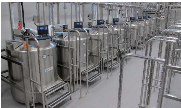
Figure 2. Cryogenic storage system. Liquid nitrogen tanks are monitored 24 hours a day and are refilled automatically.
